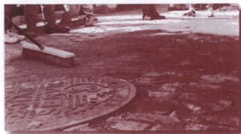
Preparing to brush in the grout (photo by Jason Swisher)
