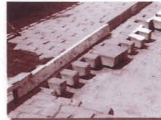
Example of "toothed" edge after removing bricks (photo by Jason Swisher)
