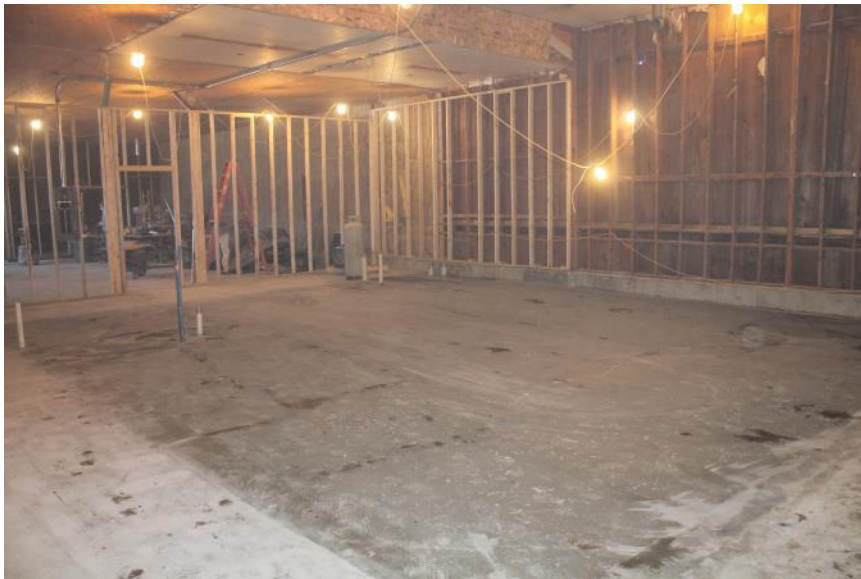
Restroom Plumbing Rough-ins
