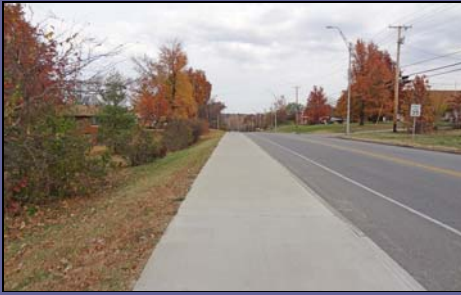
Old Hwy 63 Pedway to Stephens
